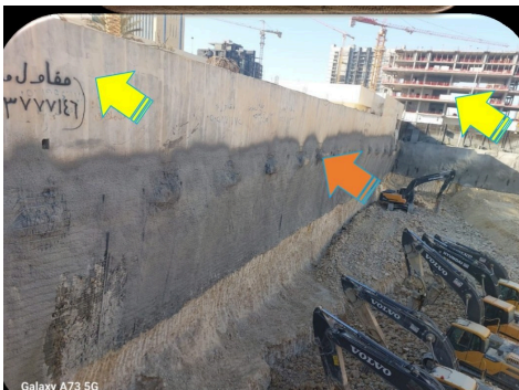
Office Tower — 4 basements, 10 floors
